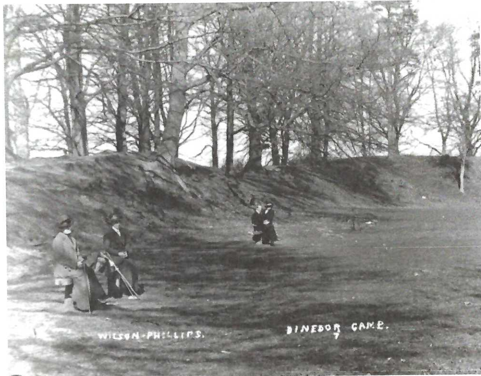
EAST END OF THE CAMP
